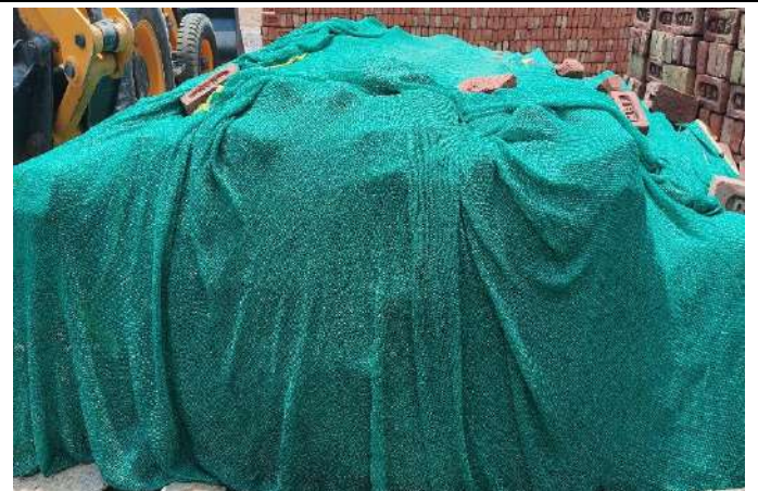
COVERED CONSTRUCTION MATERIAL
