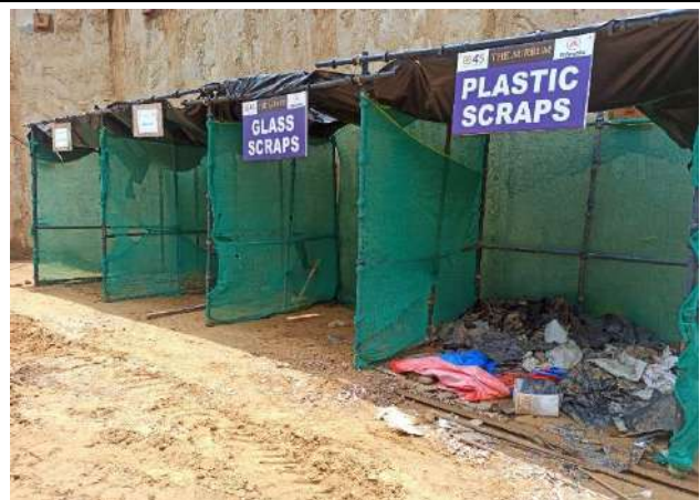
C&D WASTE SEGREGATION AREA
